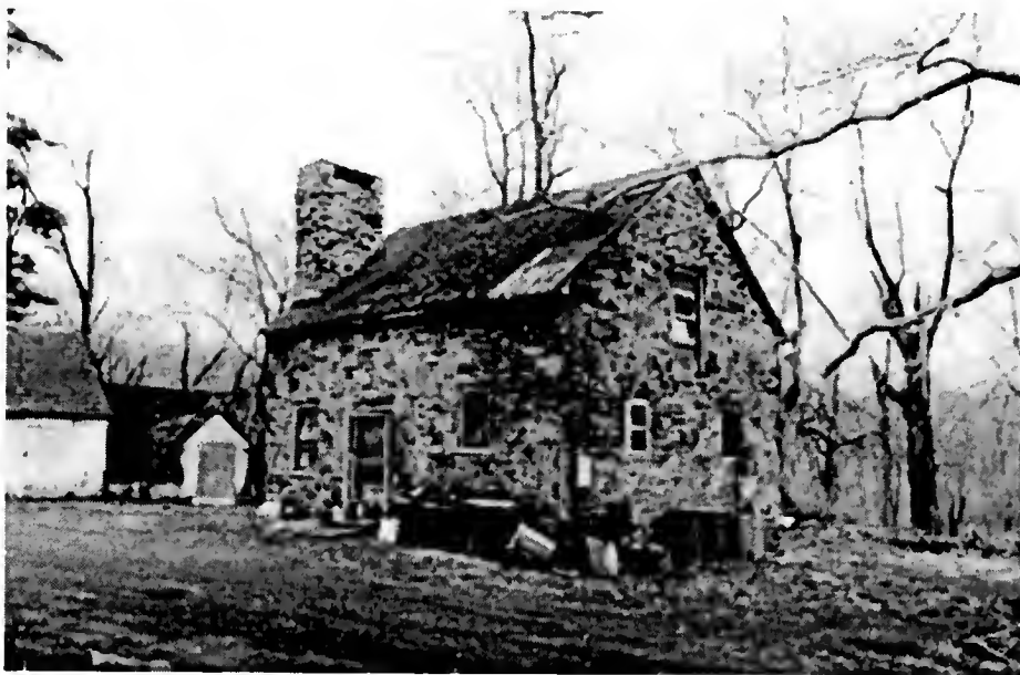
Figure 28 Caretaker’s Cottage, looking southwest, 2001
